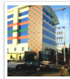
Purpose Built Office Complex at 23, Oba Akinjobi Way, Ikeja GRA, Lagos
