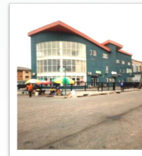
Shopping/Office Complex at 4, Salvation Road, Opebi, Lagos
